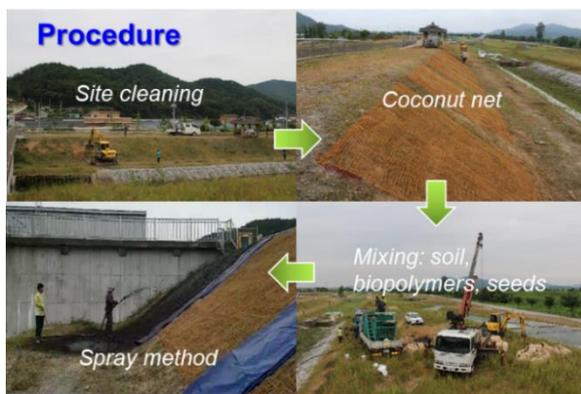
Fig. 11 Biopolymer-soil application on a cut slope
