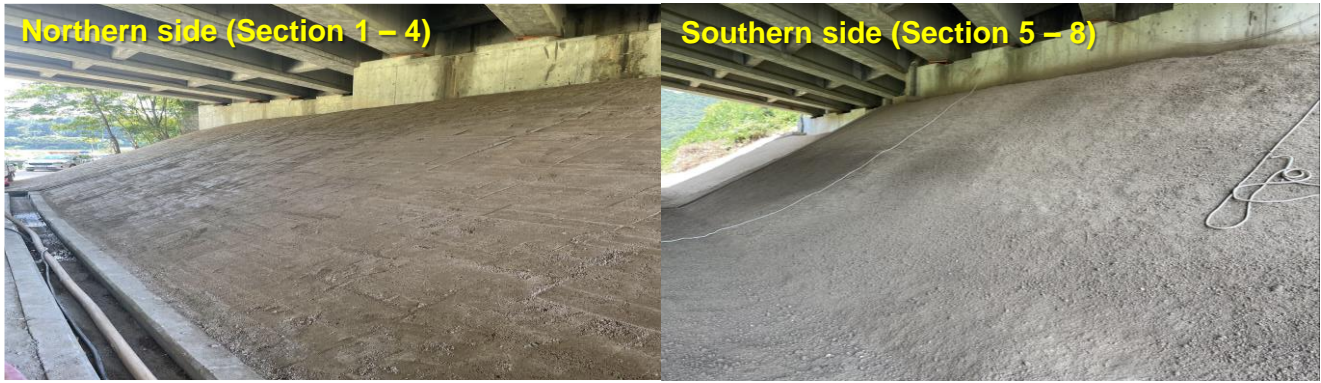
Fig. 5 Panorama view of the site after implementation
