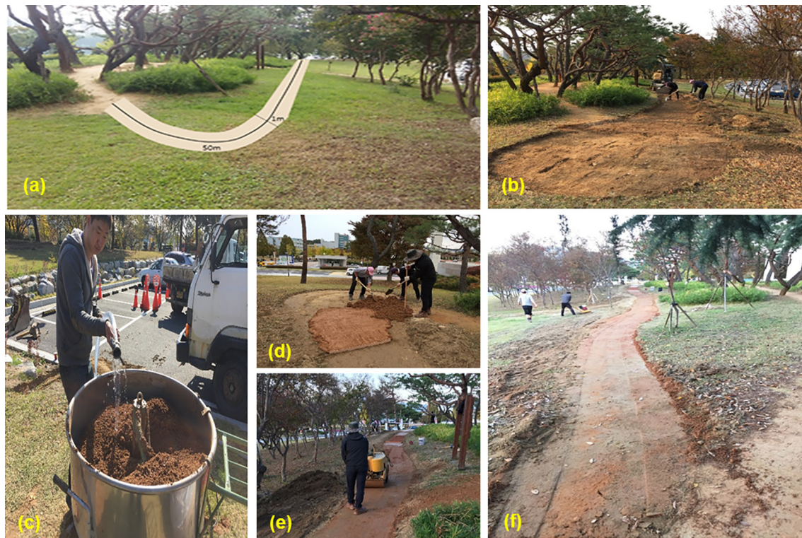
Fig. 25. Overall procedure of BPST implementation for earth surface stabilization (Daejeon, Korea; October 2015).
